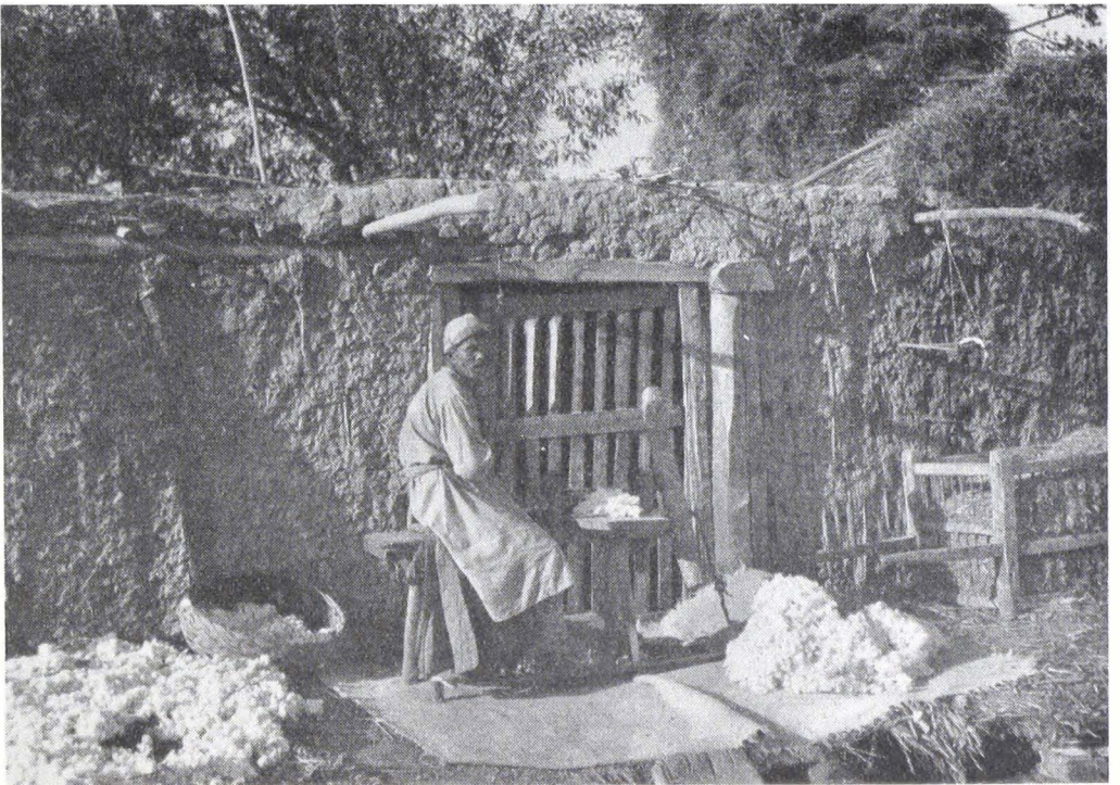
No. 4. A machine for cleaning cotton.
